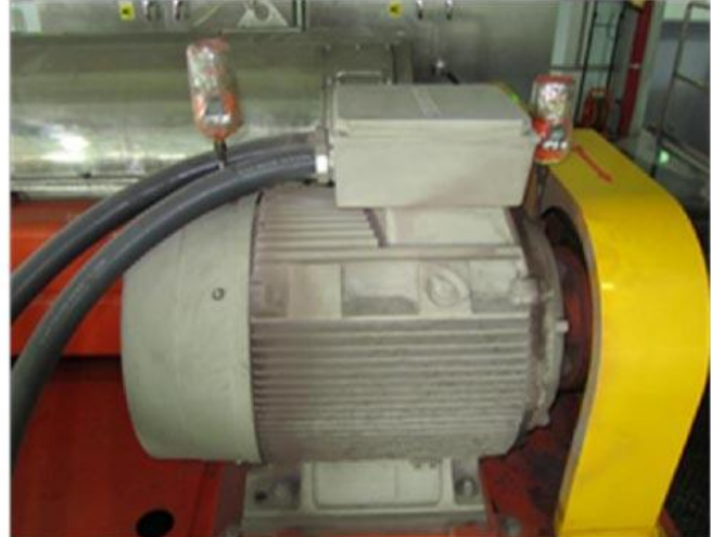
8 units of Pulsarlube M 125cc installed in Dehydration process
